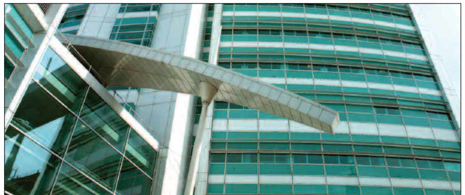
Lerch Bates supplied and installed passenger, goods, and logistics lifts, dumbwaiters, and a pneumatic tube system, as part of the integrated non-clinical support services package at University College London Hospital's new buildings.
