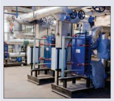
1,000-bed hospital's Lanesborough wing. Three provide heating, and two deliver domestic hot water in a duty/standby arrangement. Heating was previously provided by three shell-and-tube calorifiers, while four more provided hot water. The subsequent £45,000 savings are a combination of improved energy efficiency and reduced maintenance.
